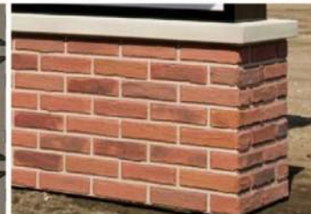
Brick Base W/ Concrete Cap
