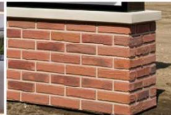
Brick Base W/ Concrete Cap
